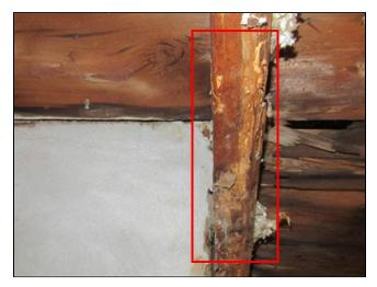
**3.7** (2) The roof sheathing was stained at the chimney. I recommend monitoring the area for further deterioration and repair as needed. The flashing at this chimney may have to be sealed or replaced.
