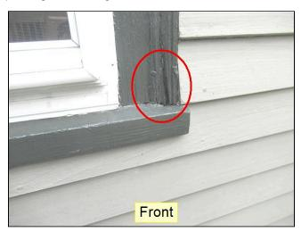
**2.0** (3) The corner board trim was decayed at the left front corner of the house. There is a potential for concealed damage behind the corner board. I recommend that this area be further inspected by a licensed contractor and repaired as needed. I also recommend the left rear corner board be secured where it's loose and any remaining gaps be caulked.
