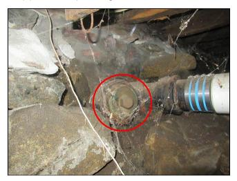
**5.4** (2) There was a leak at the first floor bathroom sink drain pop up. There was also corrosion on the bottom of the sink trap. I recommend that licensed plumber repair or replace these components.
