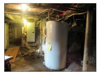
**5.7** The pressure relief valve extension on the water heater was missing. All water heaters are required to have a
