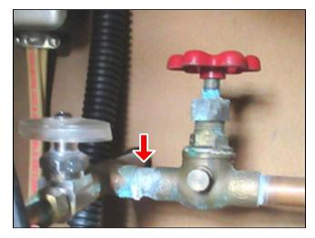
**5.1** (2) There were cut pipes in the upper kitchen cabinet adjacent to the bathroom wall. These pipes were uncapped. All cut pipes should be permanently capped. I recommend that a licensed plumber investigate further and properly cap this pipe if found to still be connected to a water source.
