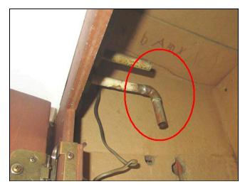
5.1 (3) There was a corroded water supply valves at the living room radiator. There is the potential for a leak at this valve. I
