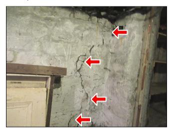
**3.0** (3) The foundation in the basement had some loose mortar. Because mortar secures the stones in the foundation, too much loose mortar can cause serious structural problems. I recommend that the foundation in the basement be prepped and re-pointed.
