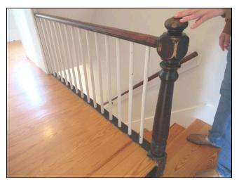
**7.2** (2) There was no hand railing at the attic stairs. All stairs with three risers or more should have a handrail. I recommend that a handrail be installed.
