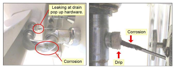
**5.4** (3) The pop-up did not operate in the second floor bathroom sink. It couldn't be opened after it was closed. I recommend that a licensed plumber repair or replace the pop-up.
