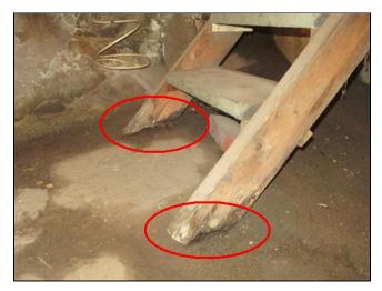
**3.1** (1) There were signs of wood destroying insect damage in the sill at the left rear and rear side of the building. Although no active insects were observed, I recommend that a full insect inspection be done by a reputable pest company.
