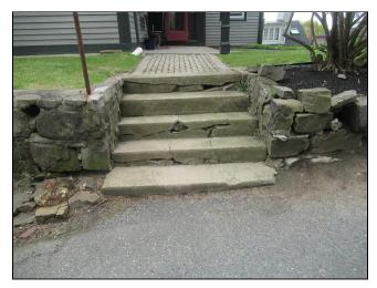
**2.6** (3) The stone steps at the front of the house are not built to current building code requirements for riser heights, tread depths and handrail requirements. I recommend caution be used when using these steps.
