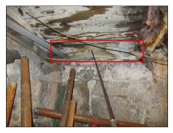
**3.2** There was wood destroying insect damage at the basement ceiling/first floor structure. There is the potential for concealed damage in the house. See previous recommendation in note 3.1.
