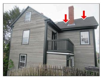
**1.3** (1) There were missing downspout extensions. Downspouts carry roof water to the ground and should have extensions that direct the water to an appropriate distance, 5 or 6 feet, from the foundation. If there are no downspout extensions, or if the extensions are too short, the roof water may eventually end up in the basement. I recommend that downspout extensions be installed to carry the water to an appropriate distance from the house.
