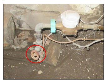
**5.1** (1) There was a corroded water supply pipe under the kitchen sink. I recommend that a licensed plumber further investigate and repair as needed.
